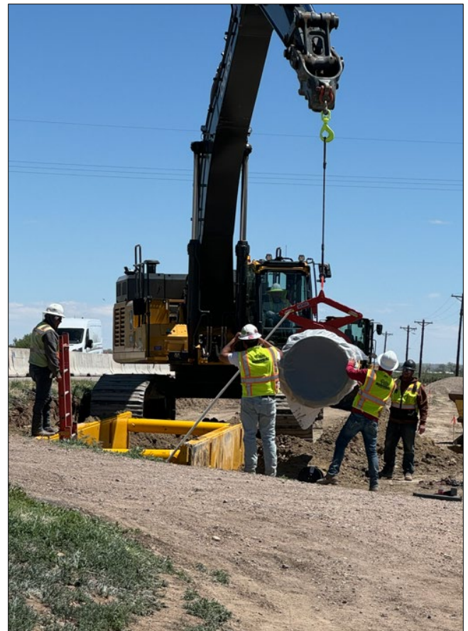
Workers for Pate Construction Company install 30-inch PVC pipe on Colorado Highway 96 as part of the Arkansas Valley Conduit Project.
